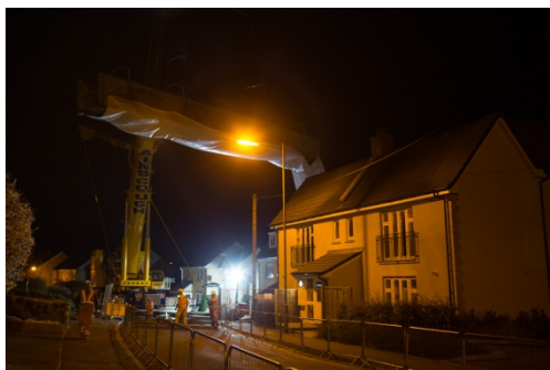
Lifting out the old bridge
