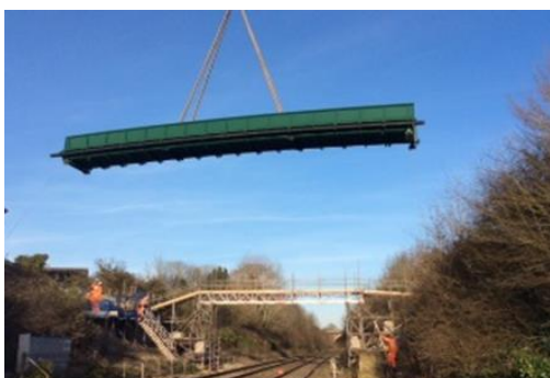
Placing the new bridge into position
